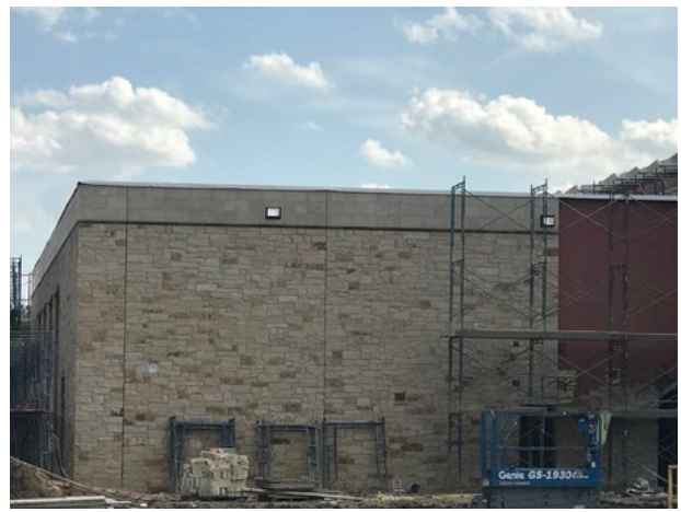
Building: Stone install on the East side
