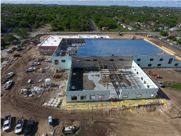
Building: Overall final 2 nd floor roof deck being installed
