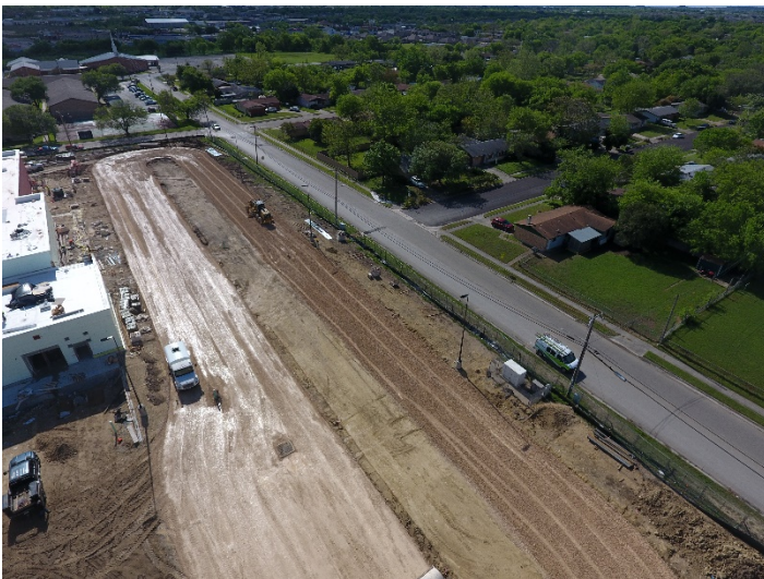
Site: South side parking lot prep work for paving.
