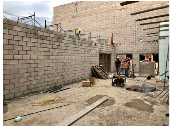
Building: CMU going up at firewalls and stairs
