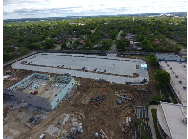
Site: Front parking lot poured.
