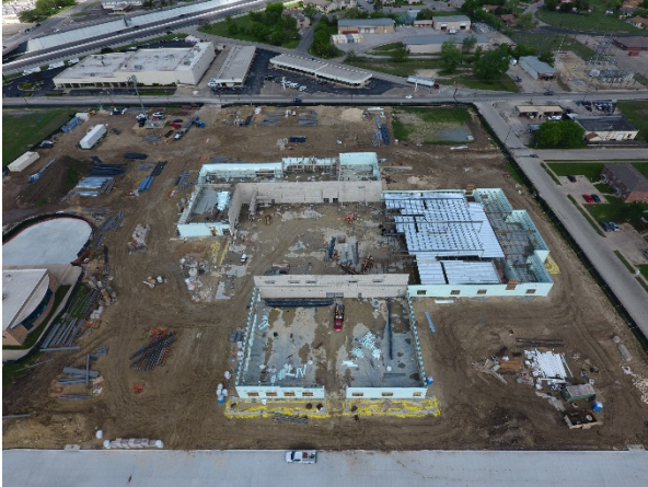
Site: First floor level of ICF framed and poured.
