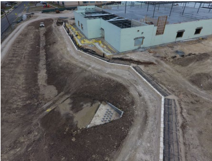
Site: Retaining wall in detention pond area.
