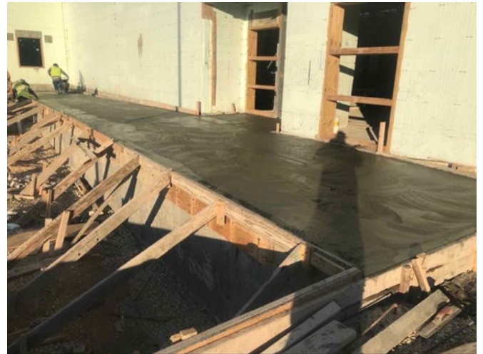
Site: Loading dock at Kitchen slab poured
