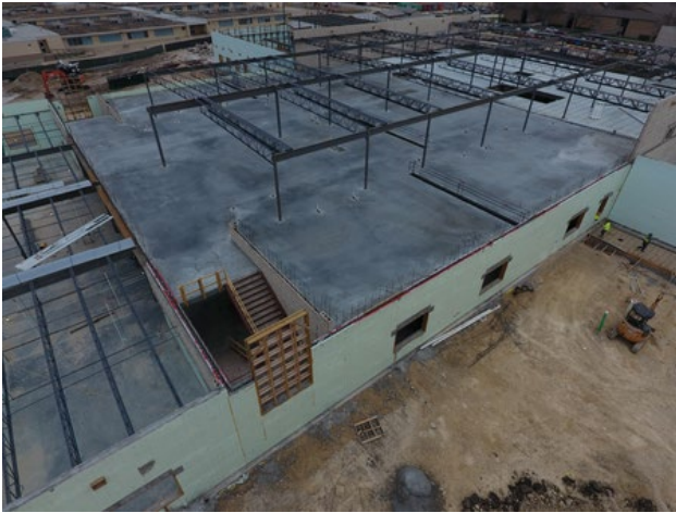
Building: 2 nd floor slab poured and framing beginning
