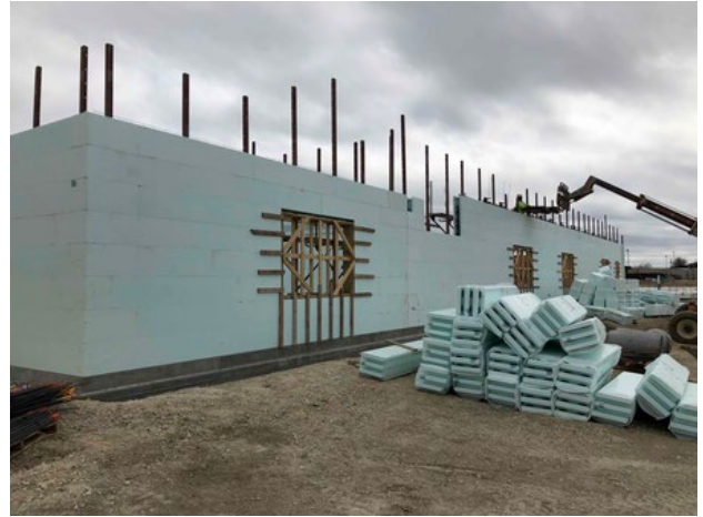
Site: Begin ICF construction area 2 & 3.
