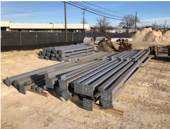
Building: Steel has arrived ready to start.
