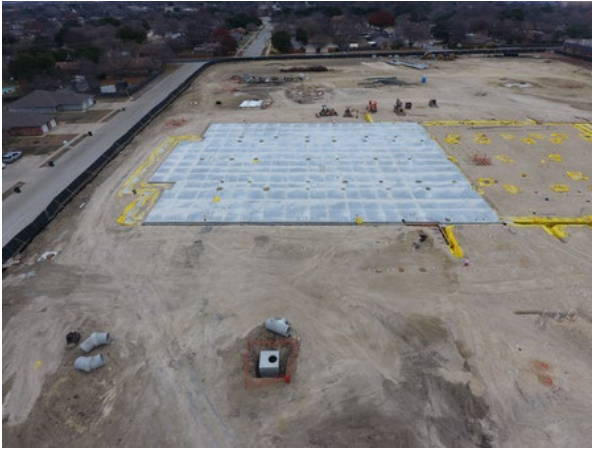
Site: Area 3 slab overview
