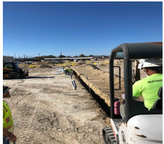
Site: Trenching for underground electric.
