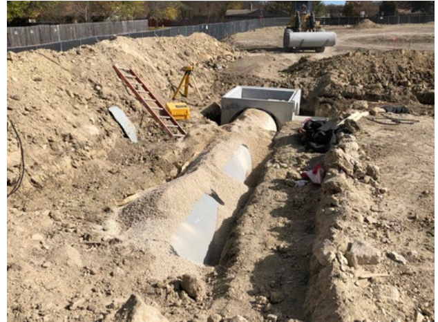
Site: Underground plumbing install
