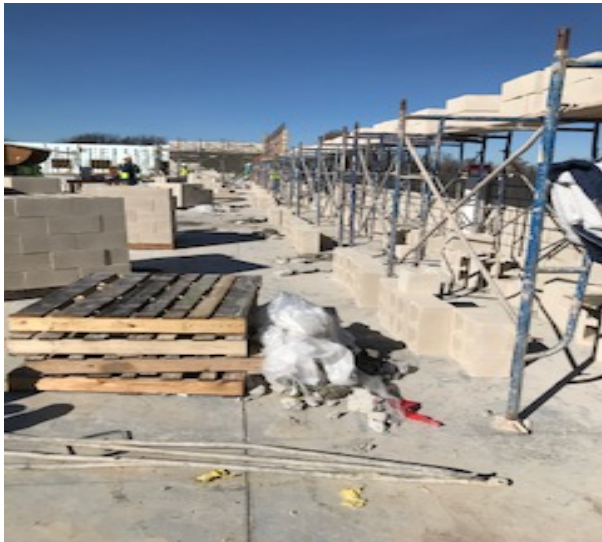
Site: CMU walls in area 2 & 3
