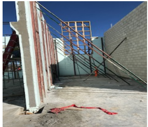
Site: Framing and walls for stairwell area 3
