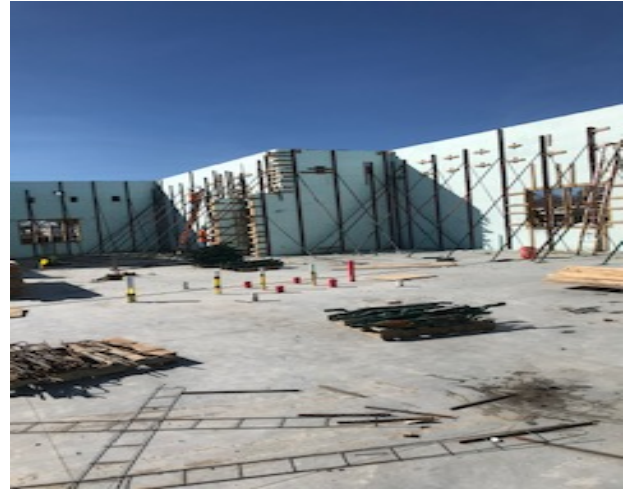
Site: ICF construction & bracing area 3
