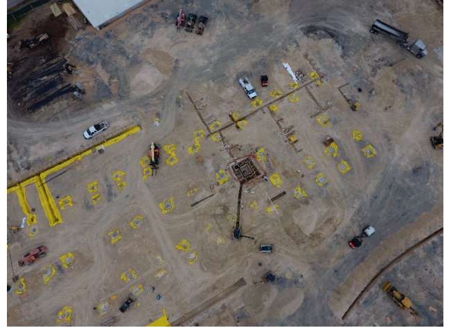
Site: Drone photos elevator pit and area 2.
