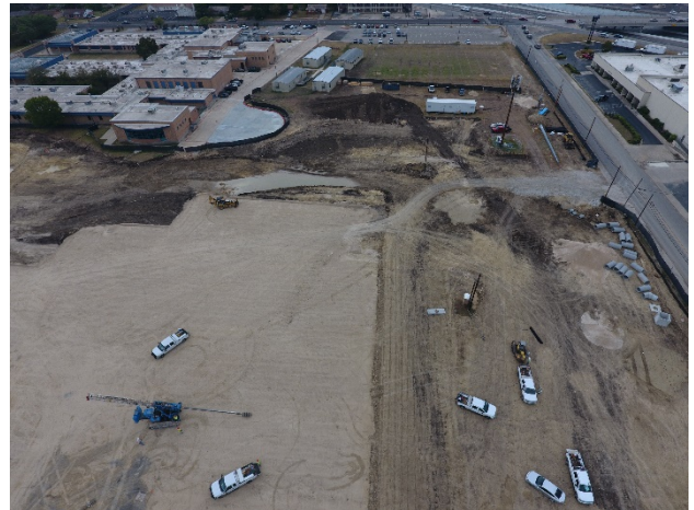
Site: Drone overview of site and pier drilling
