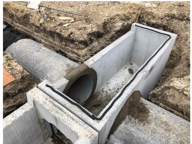
Site: Storm drain installation
