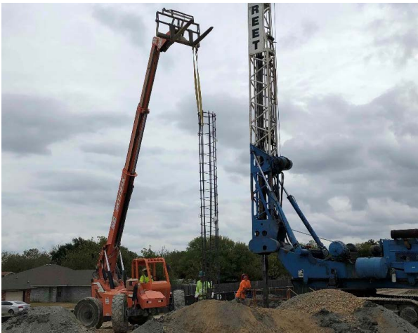
Site: Pier drilling
