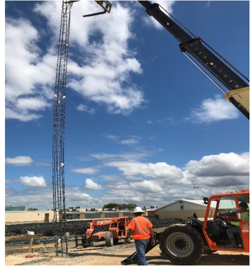
Site: Pier cages inserted.
