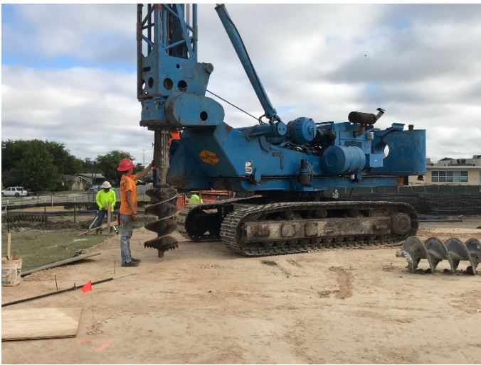
Site: Pier Drilling
