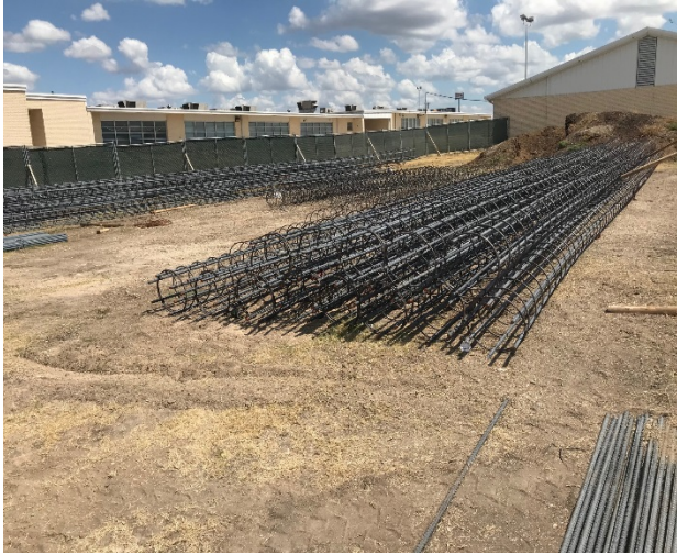
Site: Cages for piers
