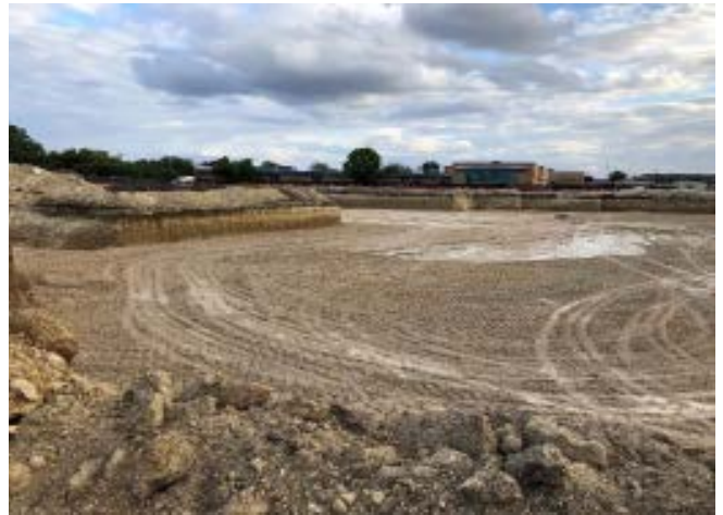
Building Pad: Looking South
