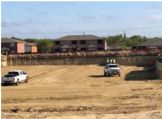
Building Pad: Looking North
