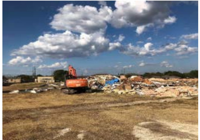
Field House: Demolition of old Field House.
