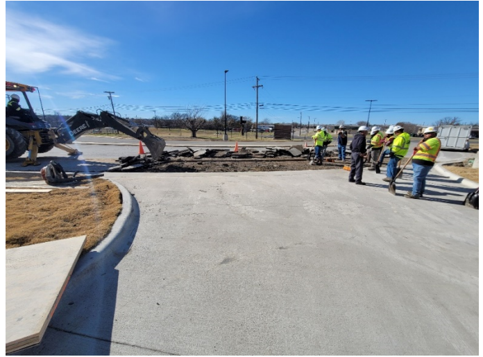
Site: Removing and replacing existing asphalt in progress.
