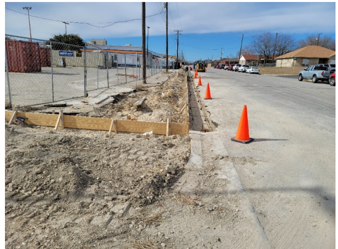
Site: Replace sidewalks at Atkinson in progress.
