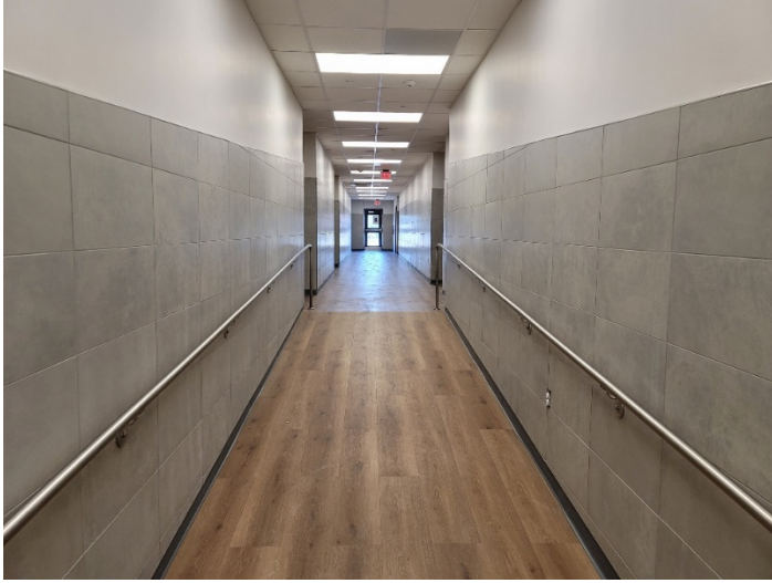
Area M: Ceiling tile, ceramic tile, base and handrail installation complete.
