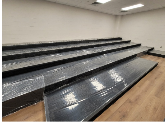
Area D: Carpet installation at platform seating complete.
