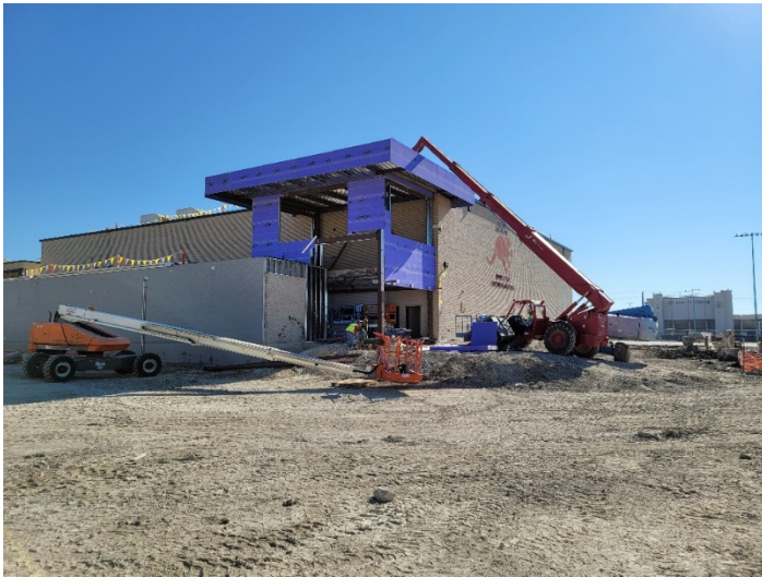
Area D: Exterior framing in progress.
