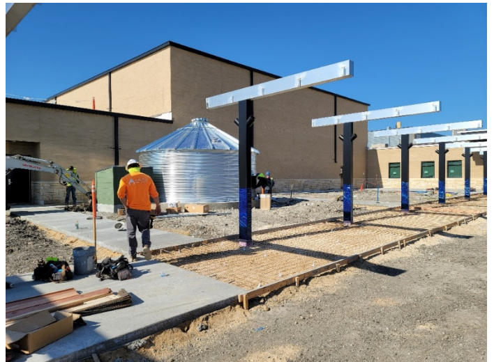
Area L&P Courtyard: Sidewalk, aluminum canopy and Cistern installation in progress.
