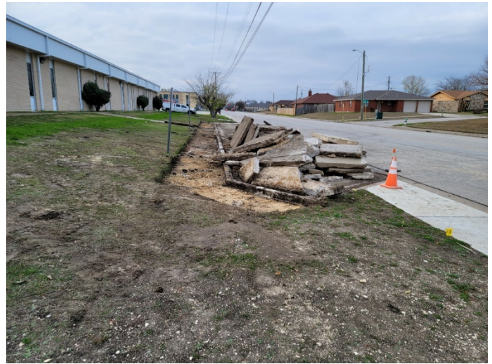
Site: Replace sidewalks at Atkinson in progress.
