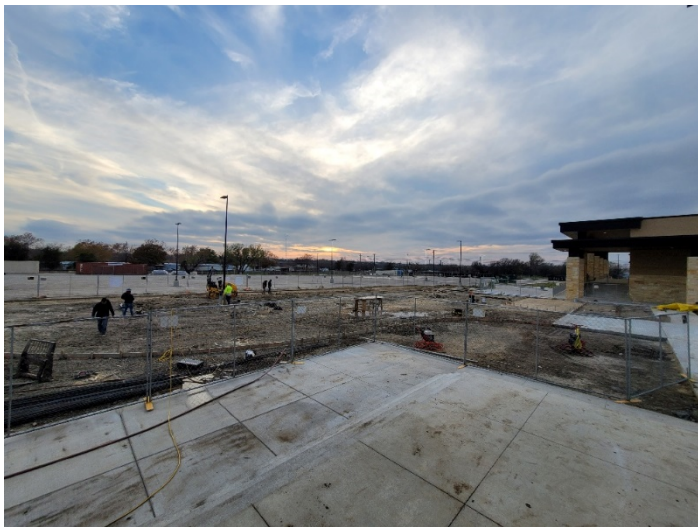
Area D&T Courtyard: Concrete flatwork installation in progress.
