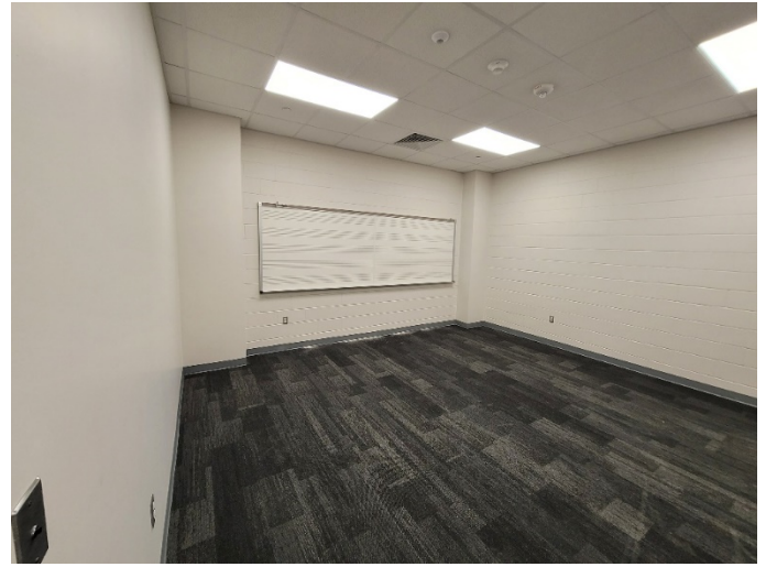
Area T: MB installation complete.
