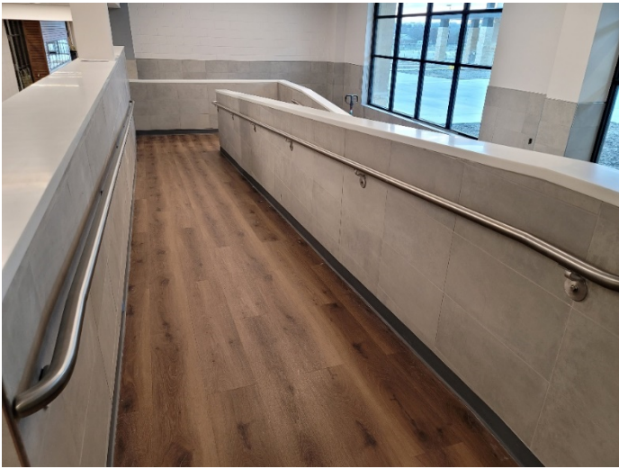
Area T: Stainless steel handrail installation complete.
