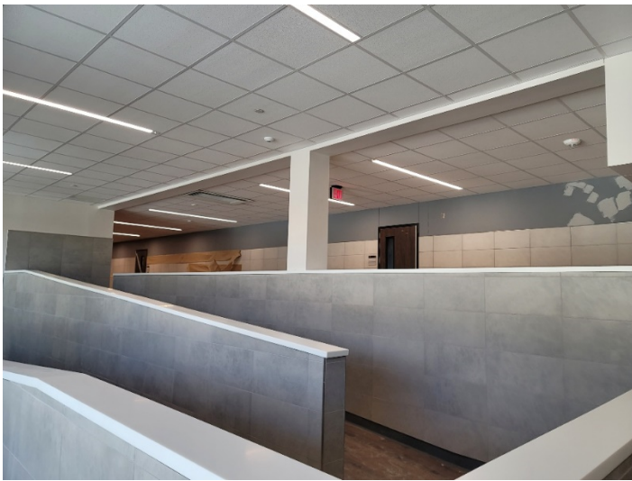
Area T: Solid surface installation complete.
