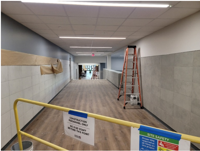
Area D: LVT and base installation complete.
