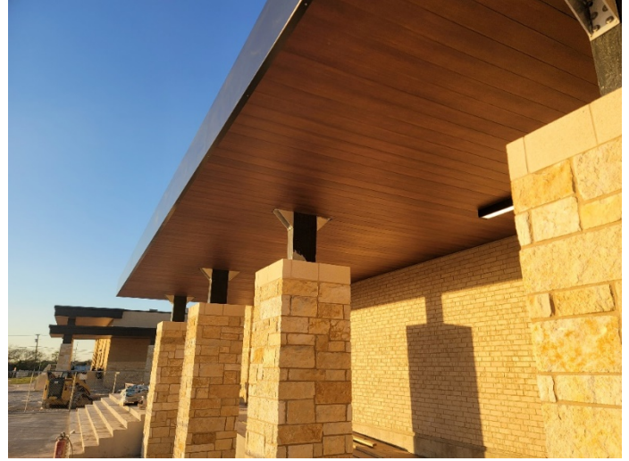
Area D: Metal soffit installation complete.
