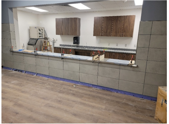
Area D: Stainless steel countertop installation in progress.
