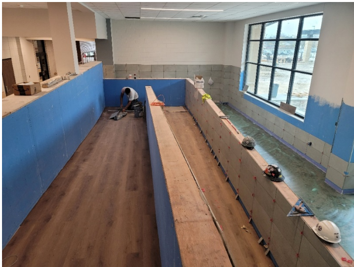
Area T: LVT and ceramic tile installation in progress.
