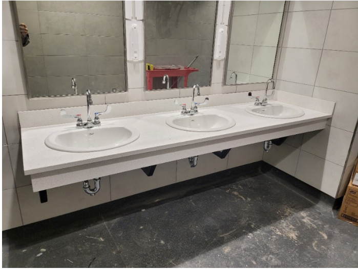
Area D: Solid surface countertop installation complete.
