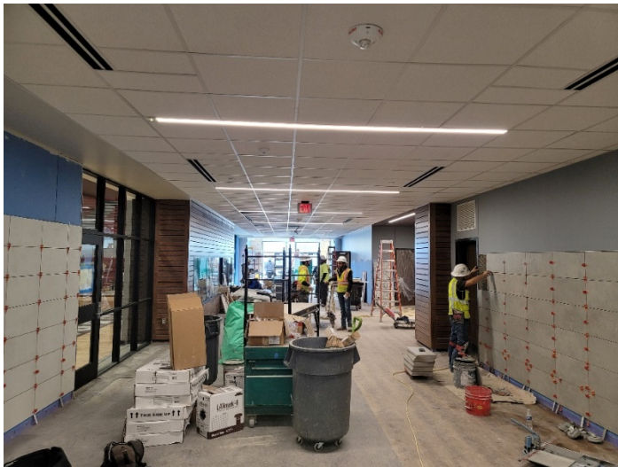
Area D: Ceiling tile installation complete.
