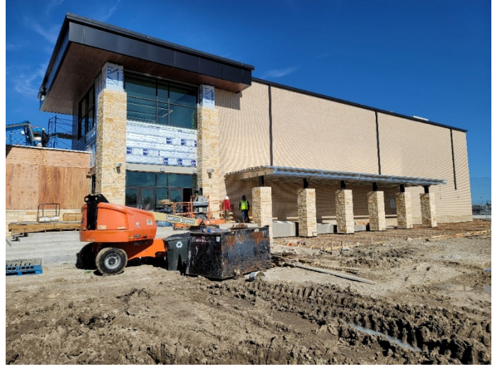
Area D: Aluminum canopy installation and concrete flatwork prep in progress.
