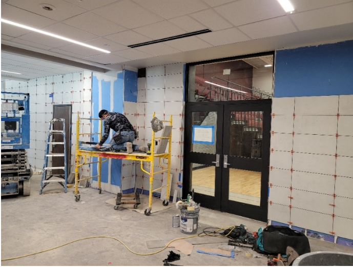
Area D: Corridor tile installation in progress.
