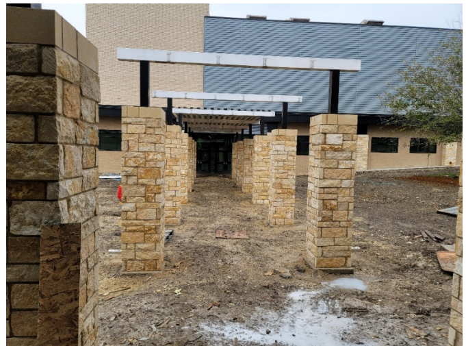
Area D&T Courtyard: Aluminum canopy installation in progress.
