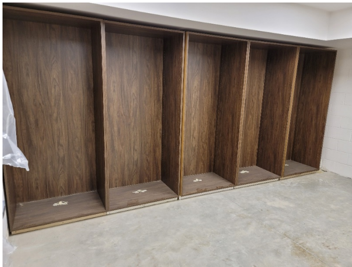
Area D: Casework installation in progress.
