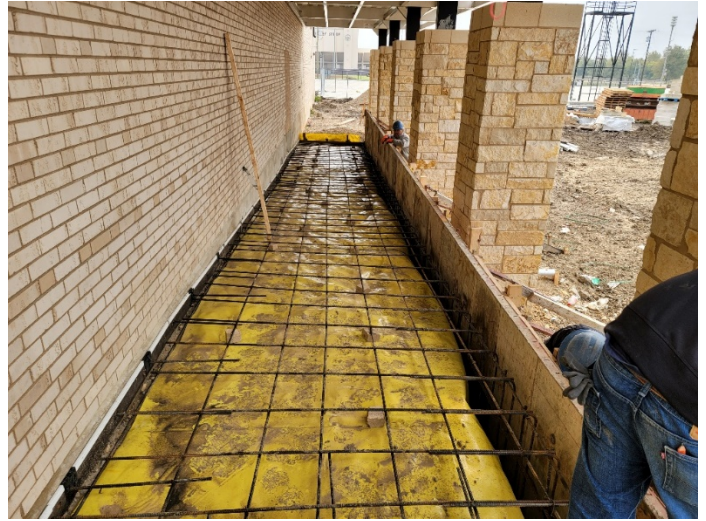
Area D: Entry ramp installation in progress.
