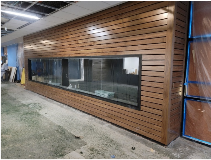
Area D: Display case installation in progress.
