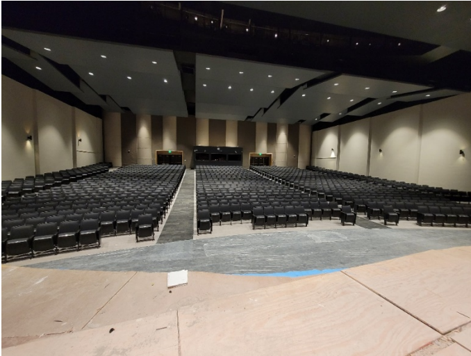
Auditorium: Seating installation complete.
