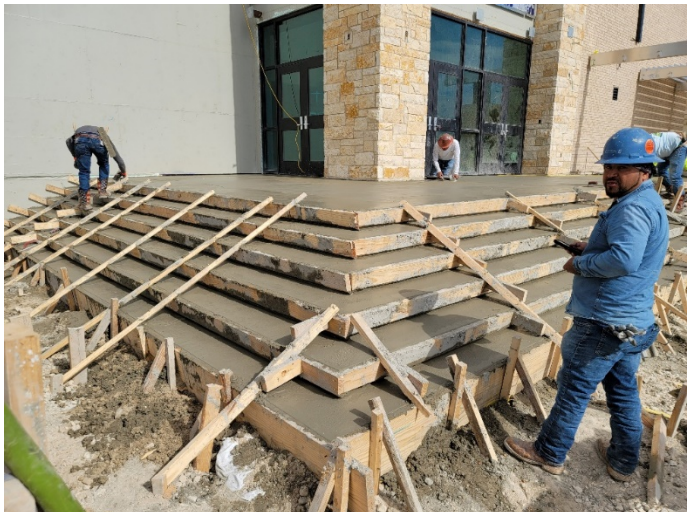
Area D: Front entry steps installation in progress.
