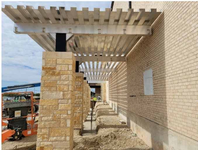
Area D: Front entry canopy installation in progress.
