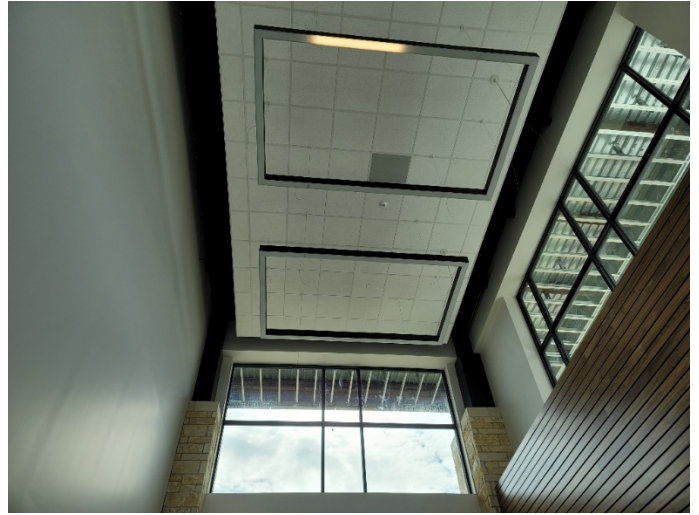
Area D: Vestibule lighting installation in progress.
