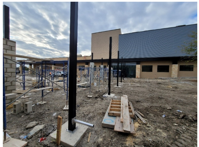
Area D Courtyard: Aluminum canopy and masonry installation in progress.
