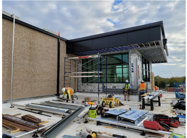
Area D: Exterior metal panel installation in progress at new vestibule.
