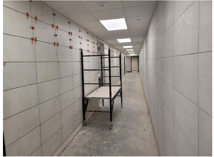
Area D: Locker room corridor tile installation in progress.
