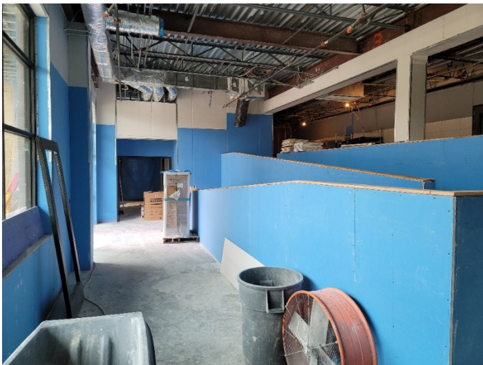
Area T: Sheetrock installation complete. Tape/float in progress.
