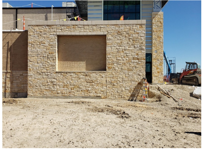
Area D & T: Stone exterior veneer complete.
