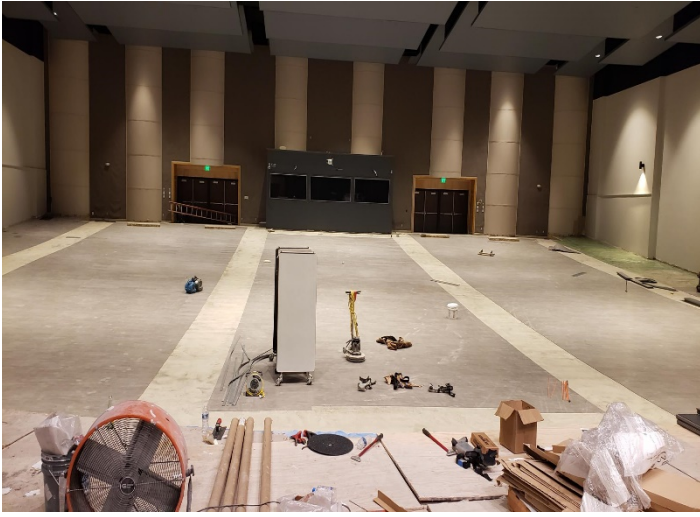
Auditorium: Flooring installation in progress.
