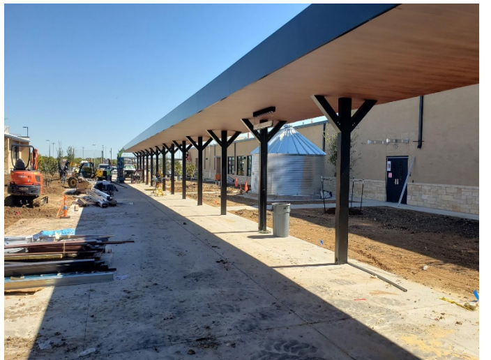
Area L&P Courtyard: Aluminum canopy facia complete. Landscaping installation in progress.
