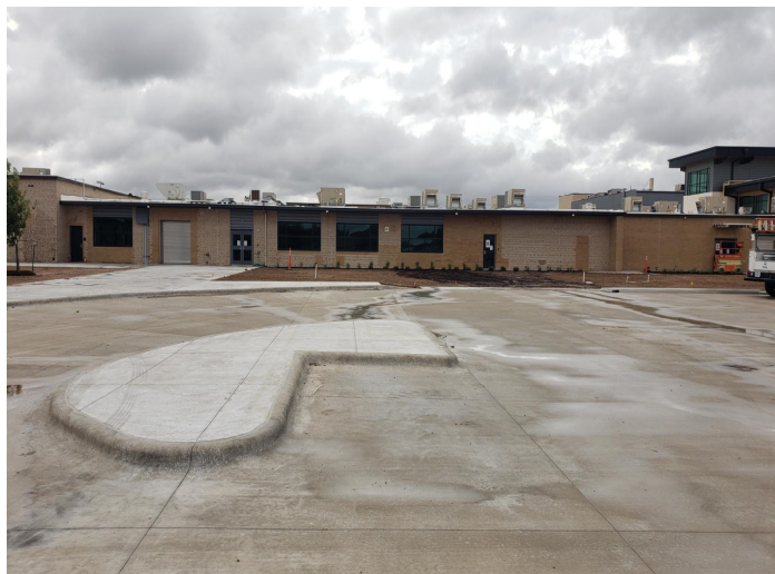
Area M & N: Aluminum canopy and landscaping installation in progress.
