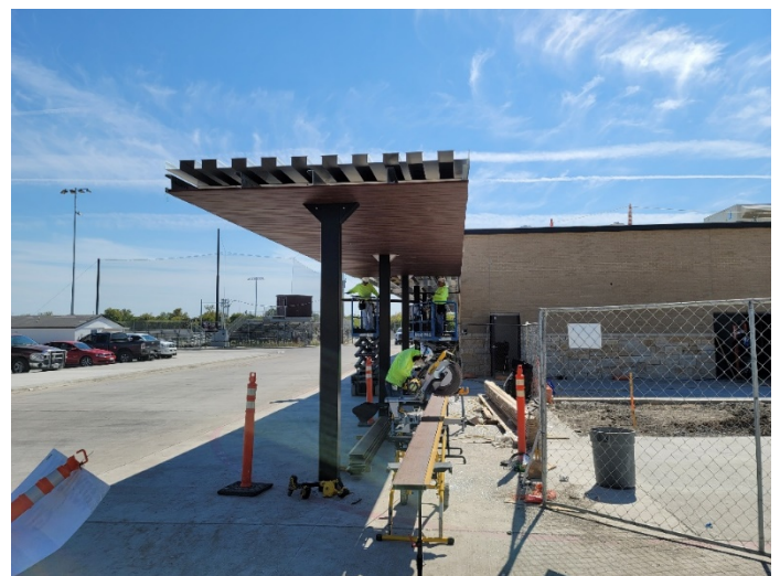
Area P: Canopy soffit installation in progress.
