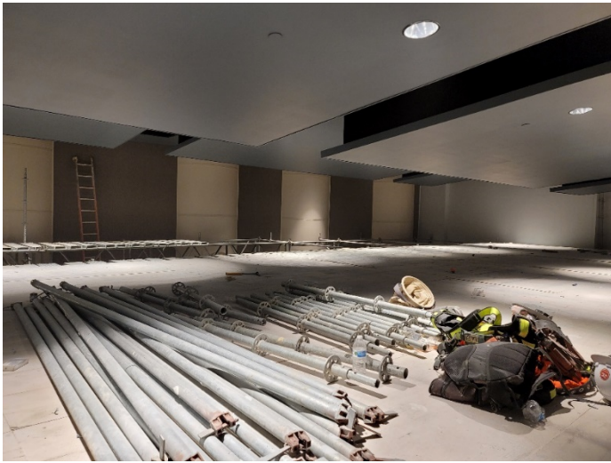
Auditorium: Scaffolding removal in progress.
