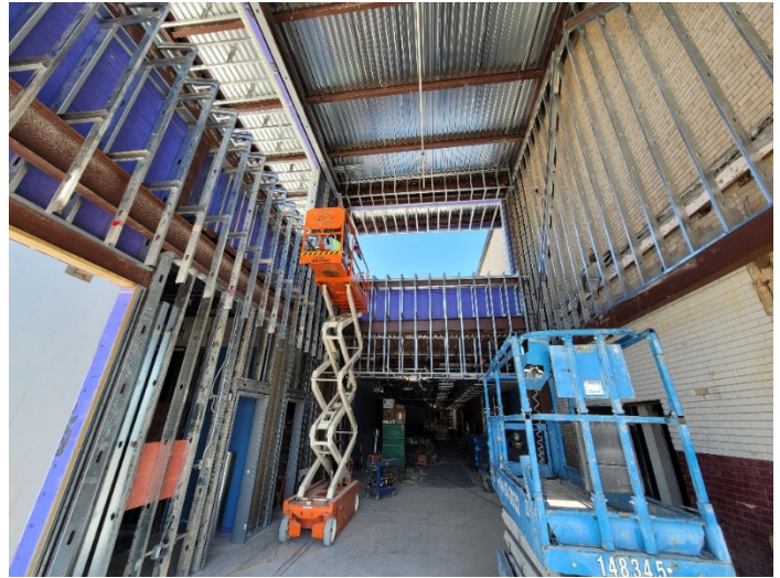
Area D: Interior framing installation in progress.
