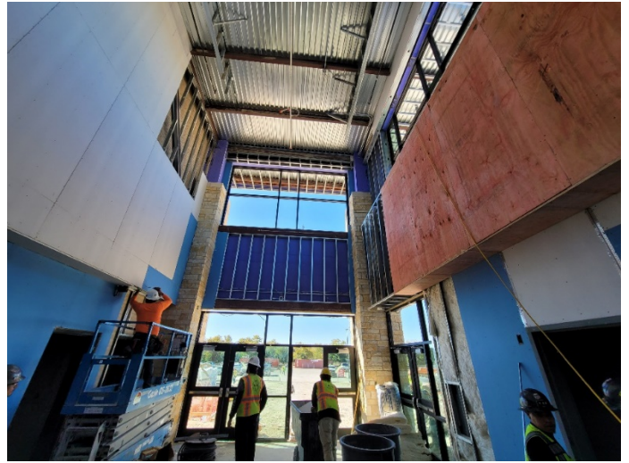
Area D: Main entry sheetrock installation in progress.
