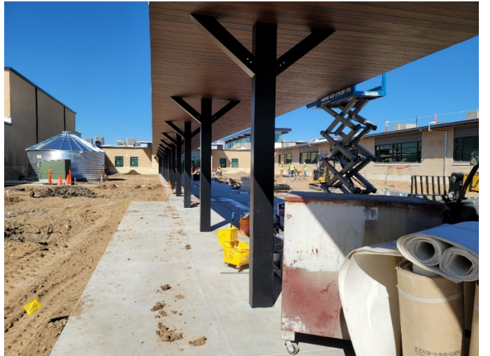
Area L&P Courtyard: Aluminum canopy soffit complete. Landscaping installation in progress.
