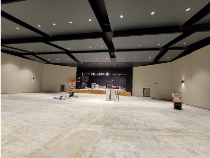
Auditorium: Wall painting in progress.
