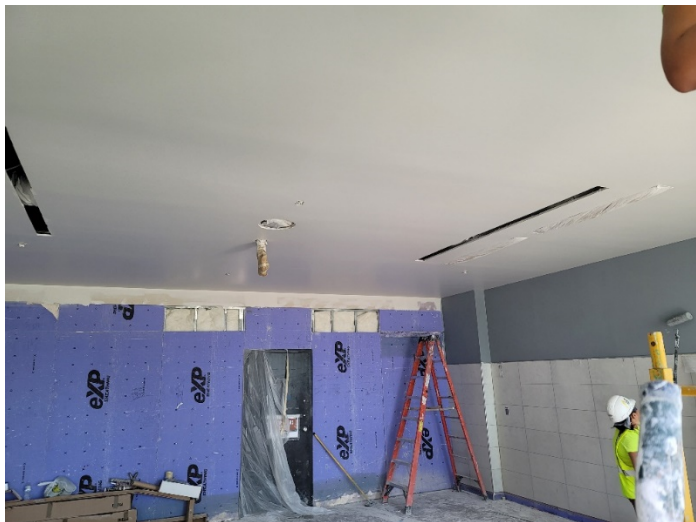
Area C: Vestibule tape/float/paint in progress.
