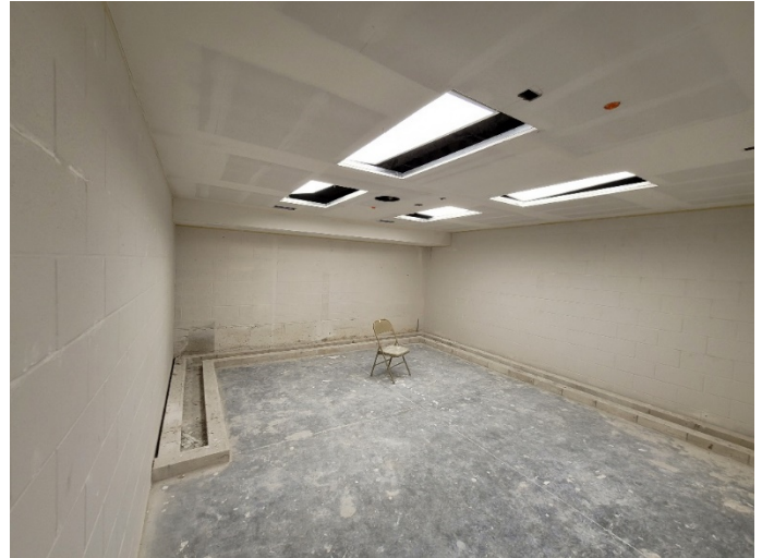
Area D: Tape/float/paint in progress.
