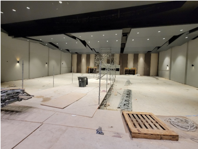
Auditorium: Scaffolding removal in progress.
