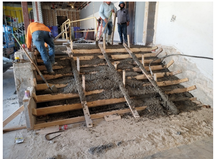
Area D: Stair concrete installation in progress.
